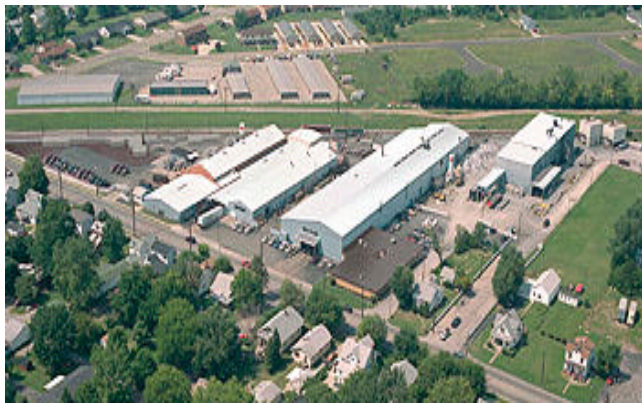
Casting - Extrusion Facility Trenton, Ohio
